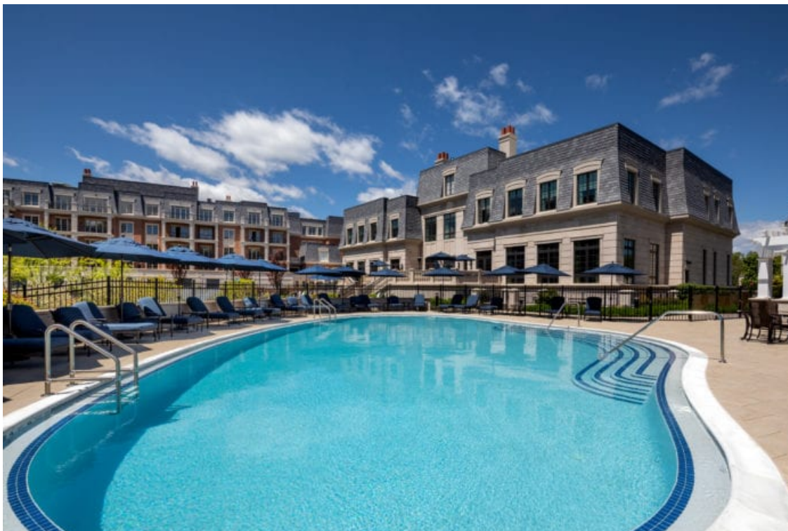
Construction at the Ritz-Carlton Residences will be complete in July. (Photo courtesy of RXR Realty)
